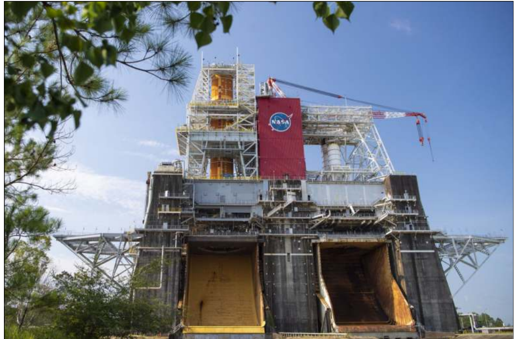
The SLS core stage is shown installed at the top left of the B-2 test stand at Stennis Space Center. NASA/Stennis photo
