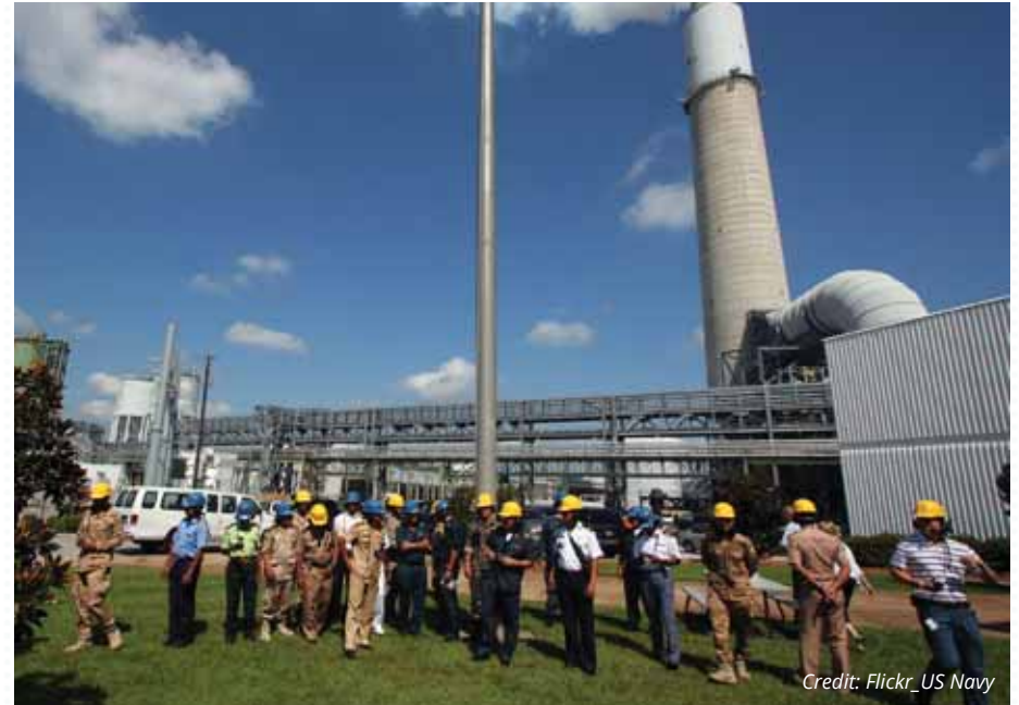
Gulf Power in Pensacola, FL.
