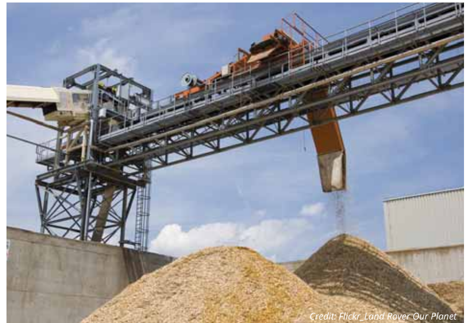
Biomass facility utilizes renewable materials to generate energy.
